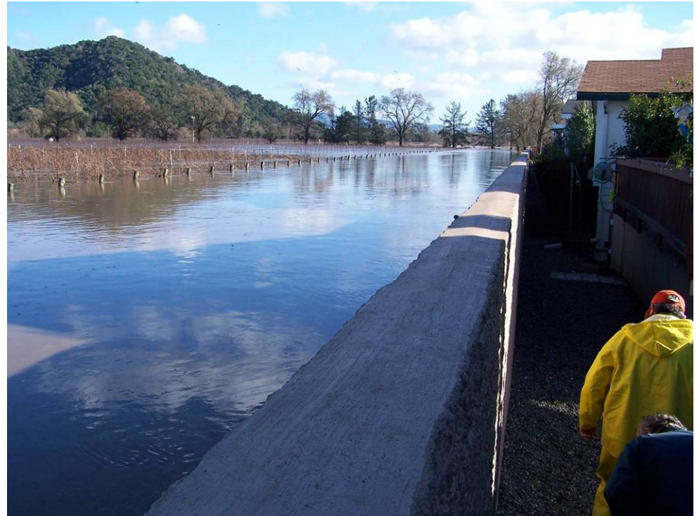
New flood wall protects previously flooded mobile homes from Napa River, 2005, Yountville, California
