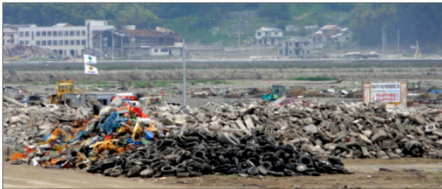
Figure 25. Separated rubber tires and concrete debris in Rikuzentakata City.
